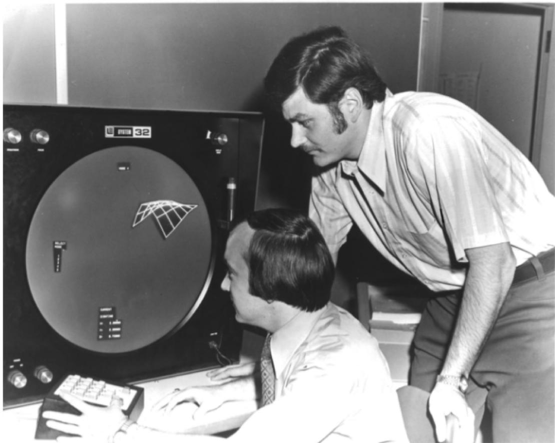
Bill Lorensen and Dick Bair (both at Watervliet Arsenal) looking at a Lundy Electronics vector refresh graphics display system. The graphics shows the results of a finite element nodal analysis.
